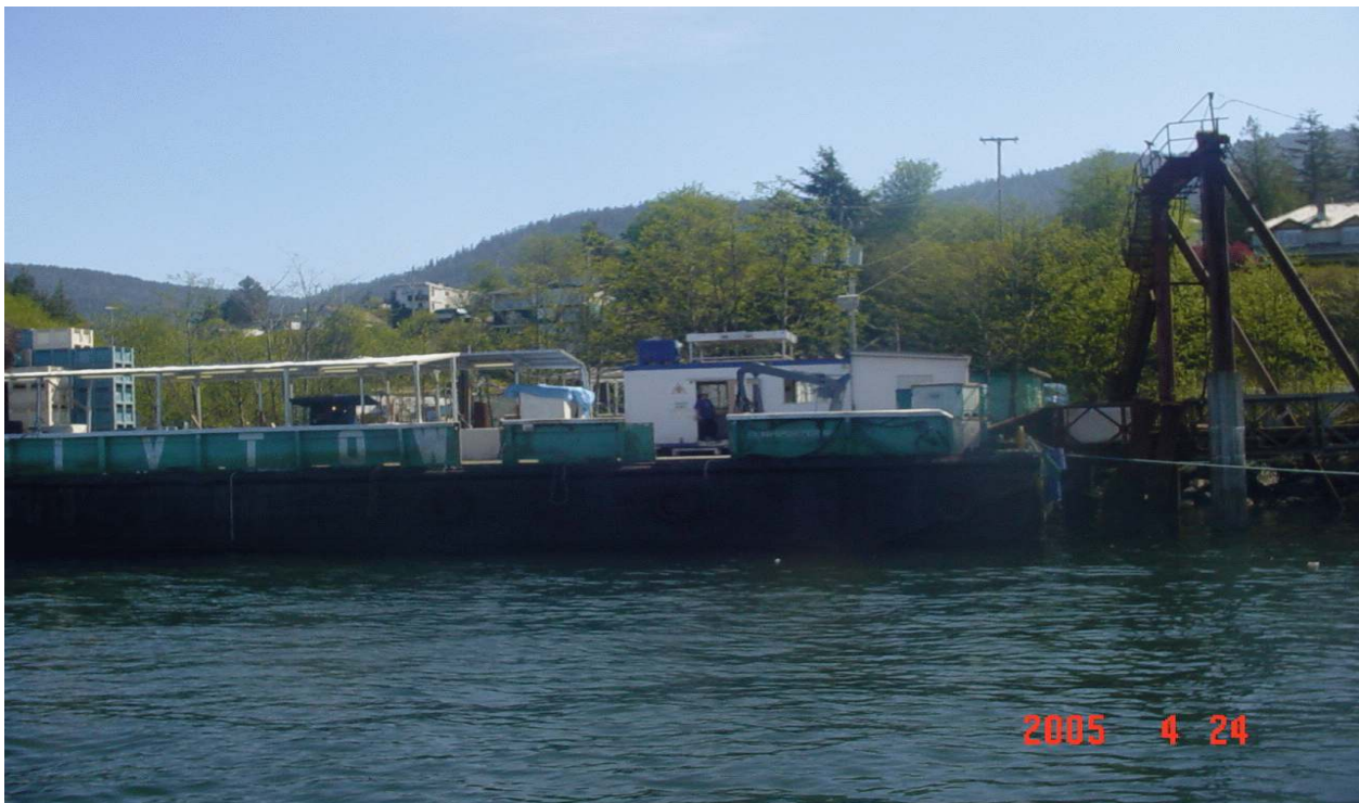
Figure 14: Keep it Cool unloading barge with entry ramp on right.
